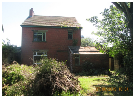
View east to the rear elevation
