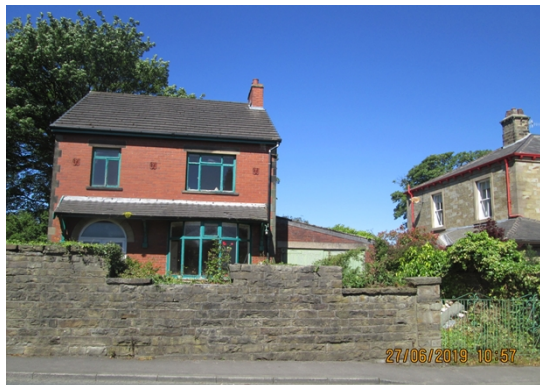
View west to the front elevation
